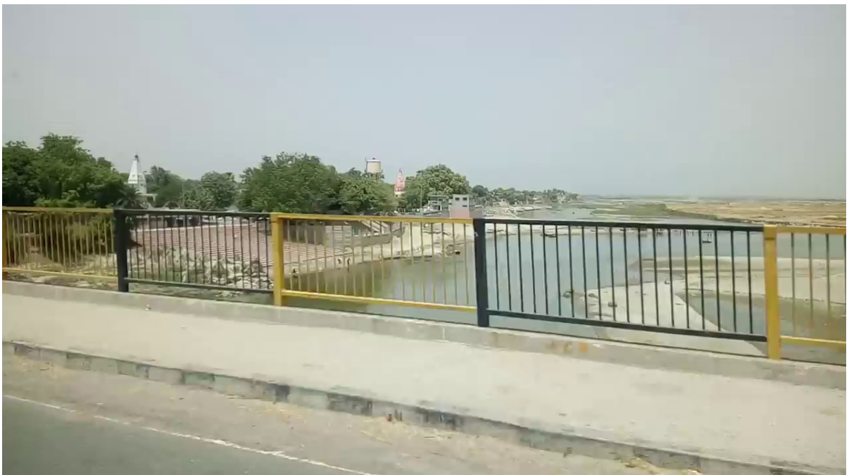
Mehndi Ghat Bridge, Ganga, Kannauj
