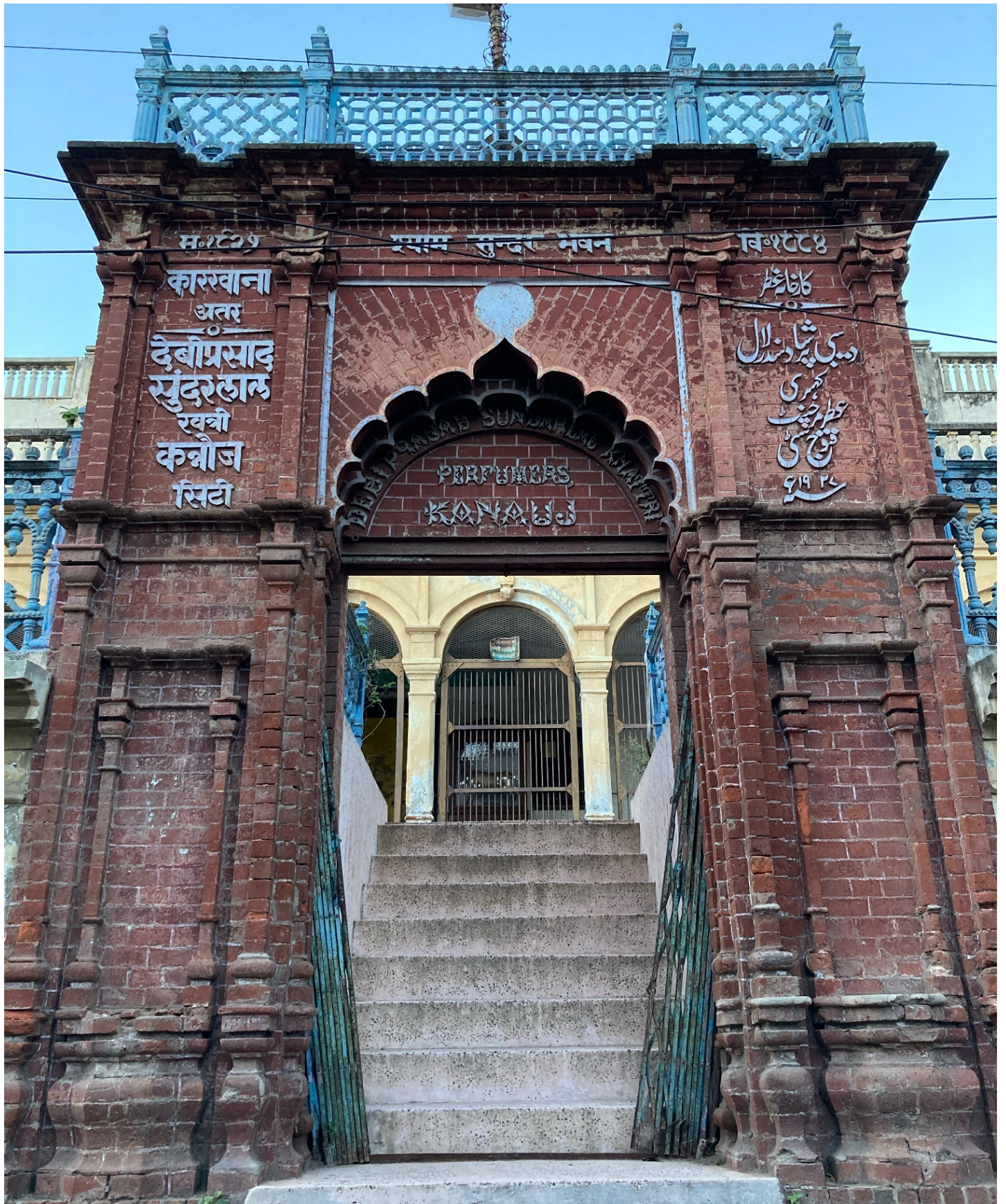
Figure 1 A beautifully constructed gate at Kannauj, Source: INTACH-ICH
